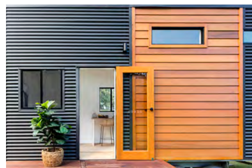
Cedar Cladding Clear penetrating oil
