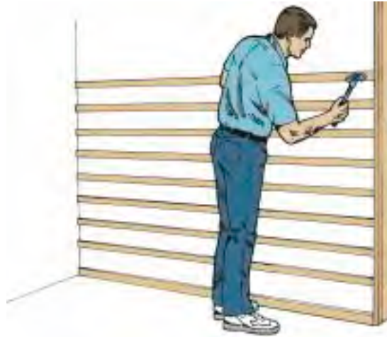
Figure 16: Furring Strip Detail
